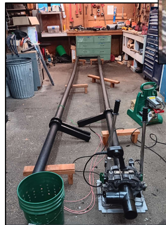
Construction of antenna array: 5 antennas 6.3 x 7-m
