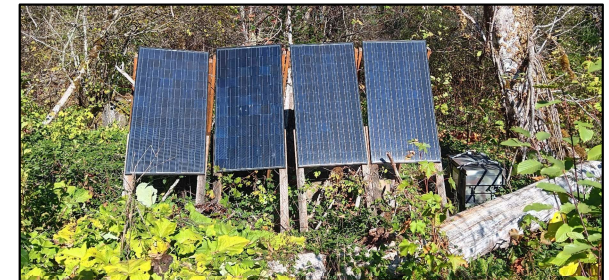
Acquisition and preparation of anchoring, electronics and power system is underway.
